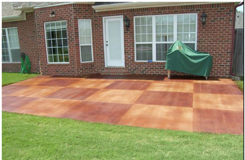
This two-color application of Color Juice Colorant and Color Juice Sealer turns an unsightly slab into an attractive patio.
